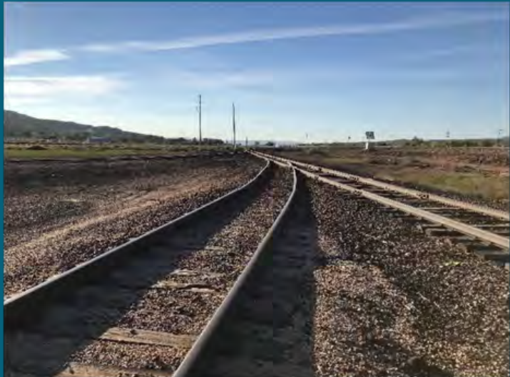
Spur (left) Splitting from Siding (right) Near Milan Industrial Park Site
