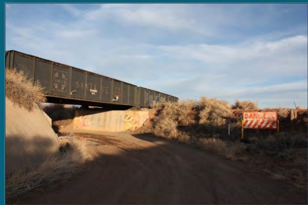
Railroad Bridge and Roadway Underpass at CR-63/Anaconda Road, Cibola County
