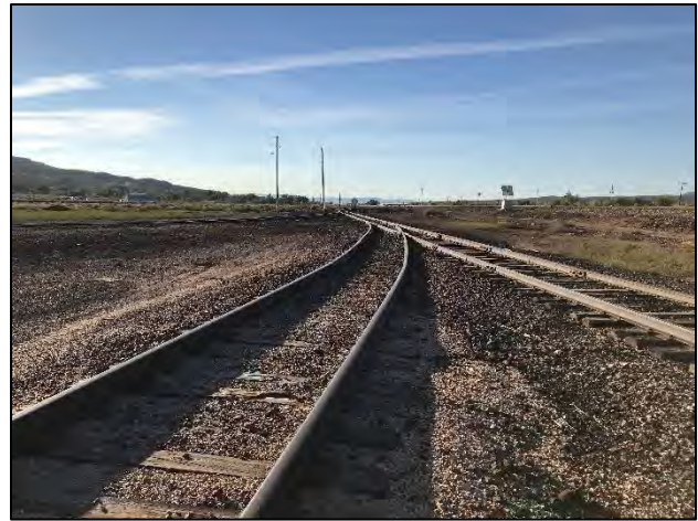
Figure 3-40: Spur (left) Splitting from Siding (right) Near Milan Industrial Park Site
