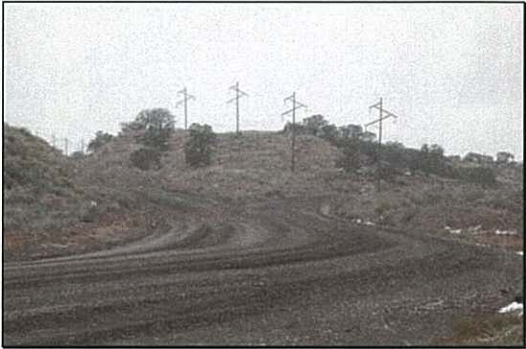
Electric Lines & Roads
