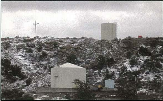
Water Tank (higher one) (50,000 gal)
