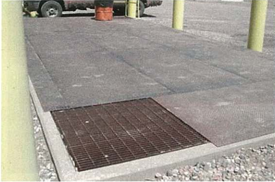
Main Office Septic Tank
