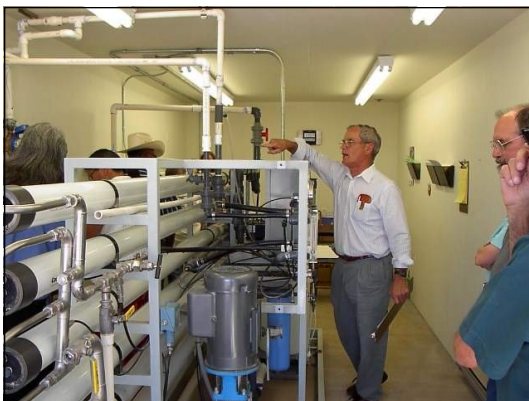
Map Above: showcases communities that participated in Phase I of the planning process. Picture to Left: Michael Daly, County Water Board Chairman, showcases a reverse osmosis system that has transformed White Cliffs MDWUA drinking water from NM's worst to best.
