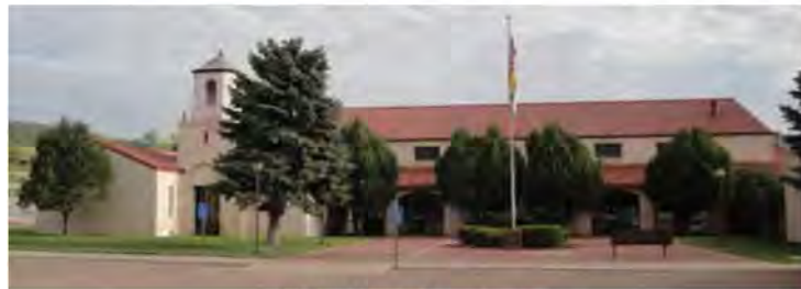
Cibola County Courthouse
